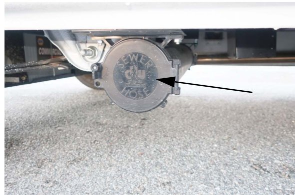
Sewage Drain Hose (Located behind the driver door area) -Typical View
